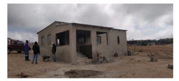
In the community of Sthobela A, near the Swaziland border, a store room structure was installed with new windows, which will help to improve ventilation. There are plans to plaster the walls soon and then to paint the outside.
